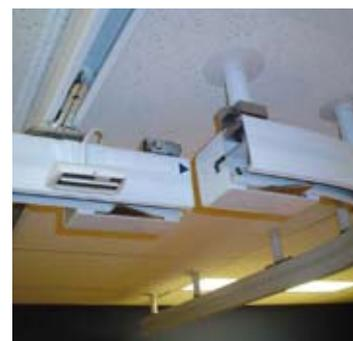
The gate, powered by *Maxi Sky<sup>600</sup>*, is a smooth way to combine a fixed track and an X-Y (traverse) system.
