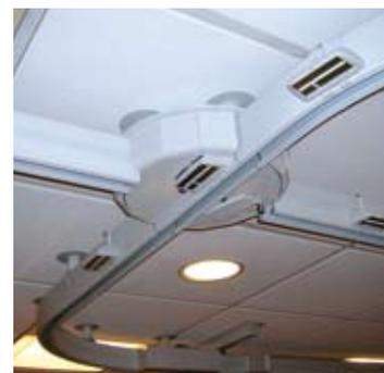
Two, three or four tracks can be connected at various angles to the turntable, which is also powered by *Maxi Sky<sup>600</sup>*.
