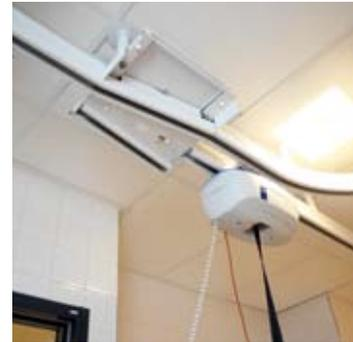
The exchanger is powered by the lift cassette of *Maxi Sky<sup>600</sup>* to facilitate track switching. This solution means no extra power supply needs to be installed.
